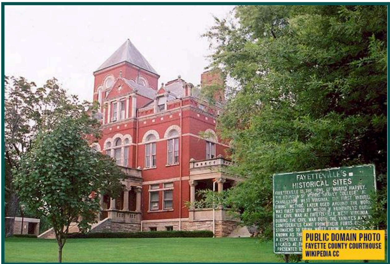
Figure 1. Fayette County Courthouse
