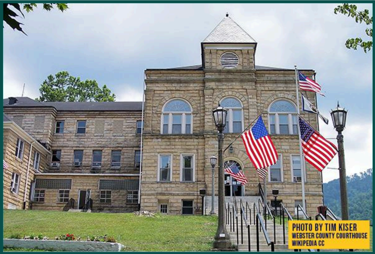
Figure 1. Webster County Courthouse
