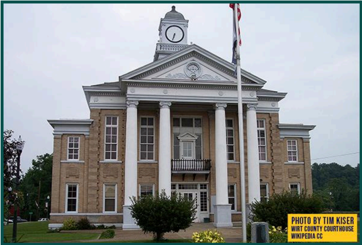
Figure 1. Wirt County Courthouse
