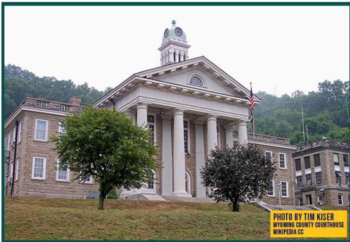
Figure 1. Wyoming County Courthouse
